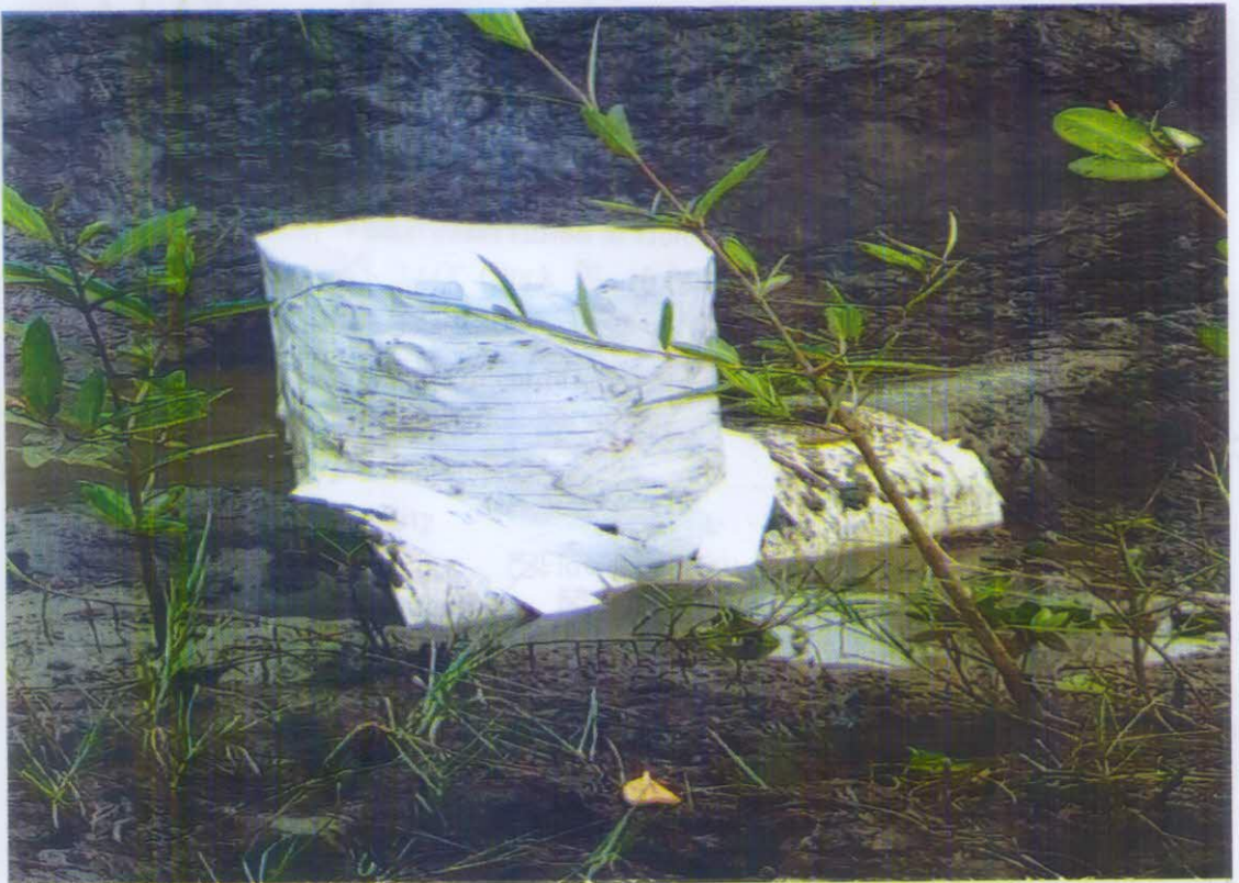
PICTURE TAKEN AFTER THE REPAIRS OF THE AFFECTED SPILLED POINT
